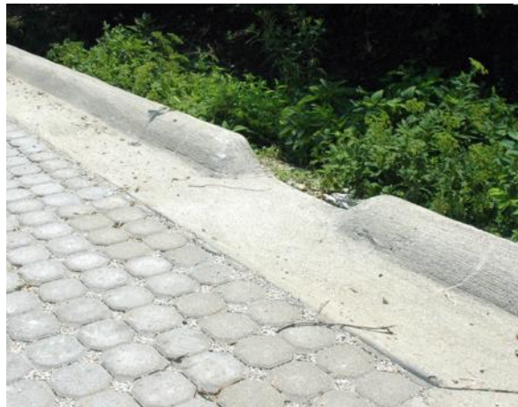
Figure 9-B: Cuts in the continuous curb allow for stormwater to be directed into landscaped areas.
