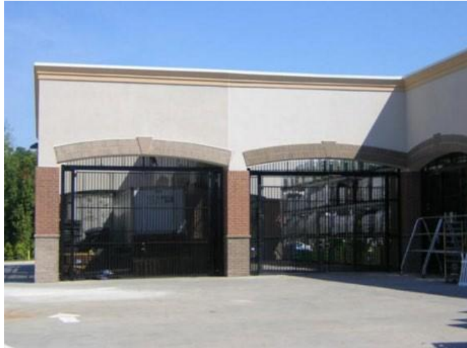
Figure 8-D: The above image illustrates a facade wall and fence that is an extension of the principal building that is designed to screen outdoor storage areas.
