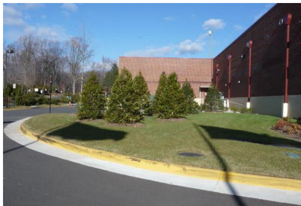
Figure 8-C: The above image illustrates a vegetative screen that hides HVAC equipment and a dumpster.
