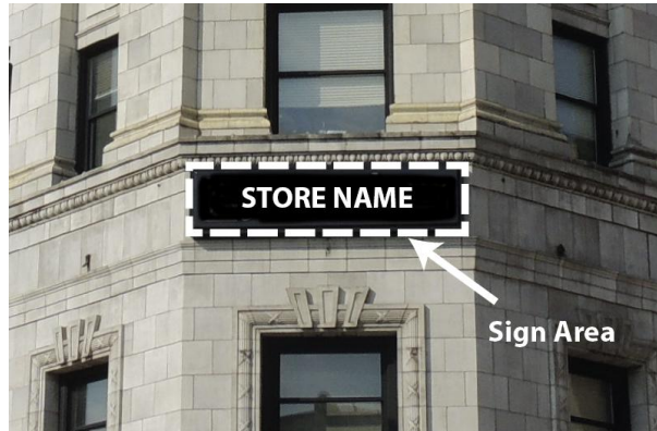
Figure 10-B: Illustration of computing the sign area for wall signs with a background panel or cabinet.
