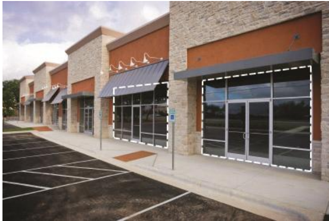
Figure 10-1: The window area is illustrated within the dashed line area for the two storefronts in the above image.
